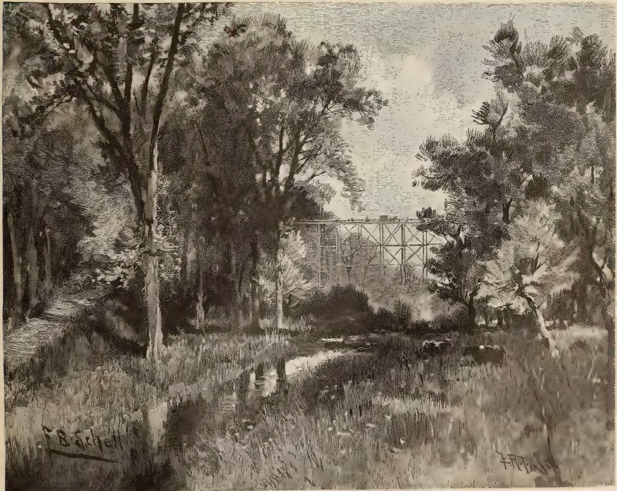
THE NORTH IRON BRIDGE, AND RAVINE, ROSEDALE.
